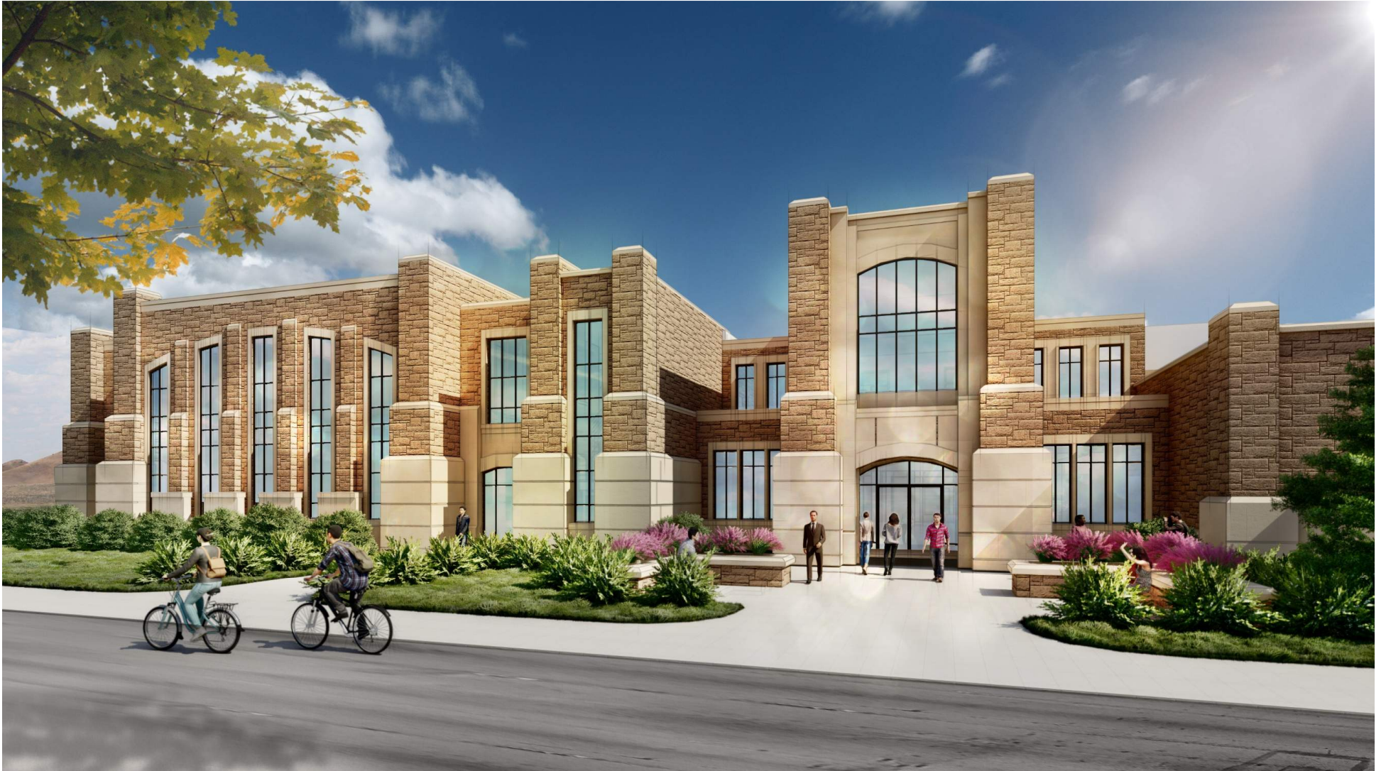
View – New Main Entry
