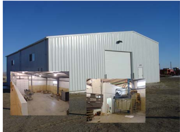
Figure 4. Inside and outside views of the foundation seed building at PREC.
