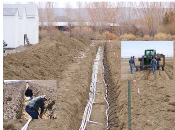
Figure 5. Sub-surface drip irrigation installation at PREC.
