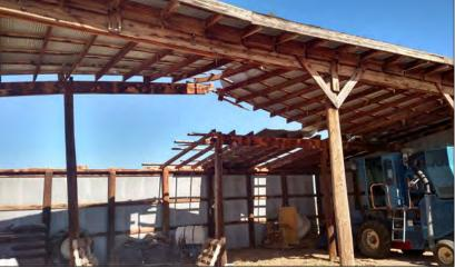
Figure 4. Shed damage from the summer 2017 windstorm.
