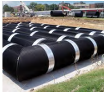
Collect Stormwater Using Appropriate Means
