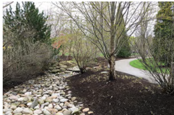
Stormwater Element – break down scale of boulders and use as a surface in stormwater BMPs and swales
