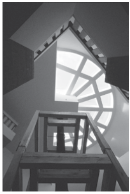
Looking up to fifth floor from the Mary Storer Loggia, American Heritage Center.
