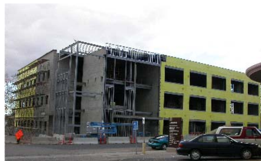
New Anthropology building, future home of the Frison Institute, under construction
