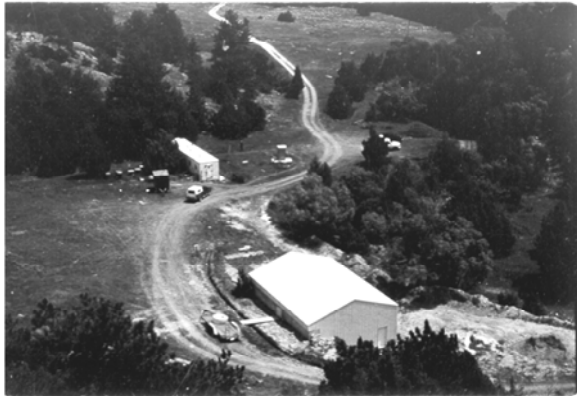
Protective Structure over Locality I of the Hell Gap Site
