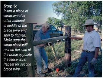
Stretch the fence from the post on the far end making sure to double wrap the wire around the post at the start and end of the run. A staple on each wire will help hold it in place and assists in stretching the fence.
