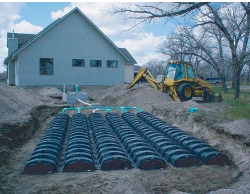
*Conventional gravity fed septic system with concrete tank and distribution box. The drain field is a bed configuration with chambers that do not contain gravel.*
