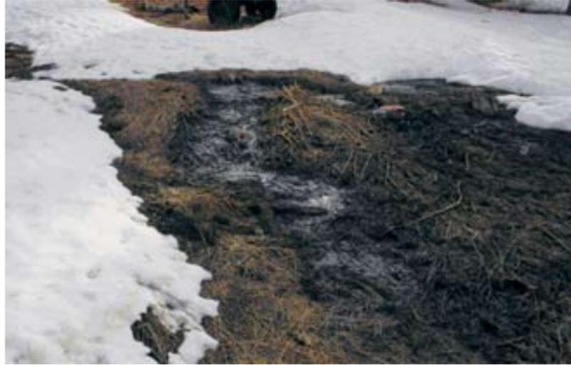
*Effluent can be commonly seen surfacing in the area when a drain field fails.*
