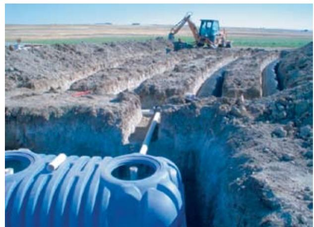
*Gravity fed system in a trench configuration. A plastic (poly) tank and distribution box are used with this system.*
