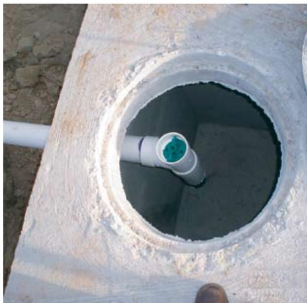
*This is a picture of the outlet baffle in a concrete tank. The green object inside the baffle is an effluent filter that must be removed and cleaned at least every six months. The effluent filter keeps solid material from entering the drainfield.*
