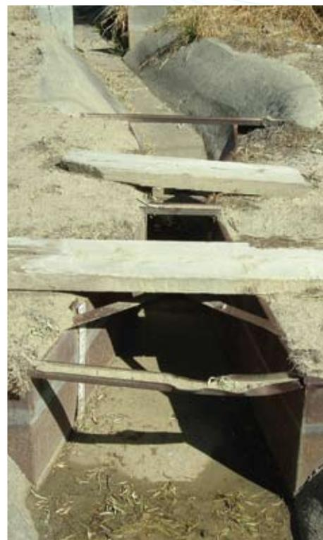
*A simple concrete weir with gauge measures water flow.*
