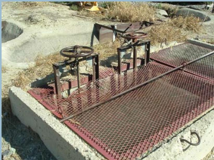
*A head gate controls release of water from a supply ditch.*
