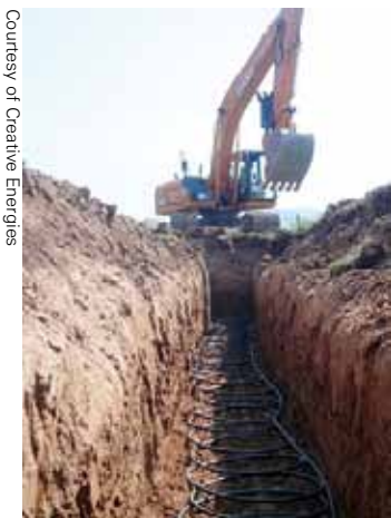
This small residential geothermal loopfield using a single slinky coil in a trench requires the disturbance of existing landscaping and adequate space. (Driggs, Idaho)
