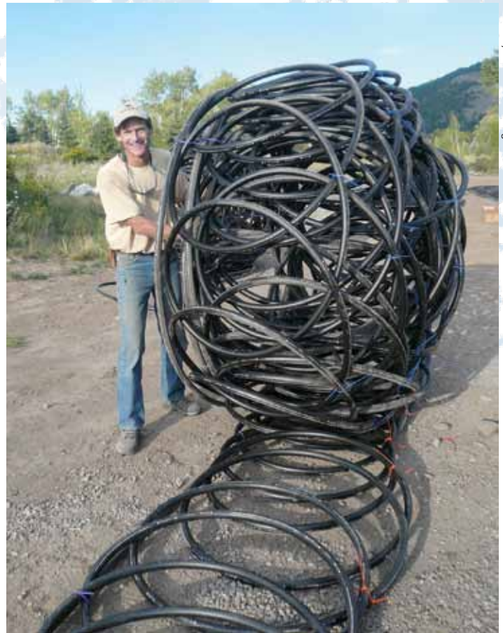
Building the loopfield in a pit or trench is sometimes impractical. In those cases, the coil is pre-assembled, rolled into an orb, and unrolled in the pit. (Jackson, Wyoming)
