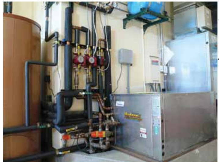
A finished heat pump system utilizing a water-to-water heat pump, a water-to-air heat pump, and a buffer (pressure) tank (left). (Jackson, Wyoming)
