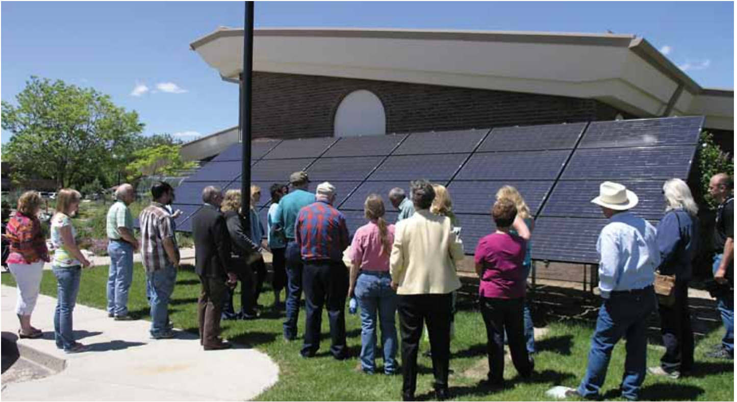
The UW Cooperative Extension Service wind/solar demonstration system at the Natrona County Agricultural Resource and Learning Center offers Wyomingites a chance to see how both an on-grid and battery-based system function. The 4.2 kW solar array technically allows one of the offices in the building to be "off-grid." The system was completed with UW CES, UW School of Energy Resources, Natrona County, and Rocky Mountain Power Blue Sky Program funding.
