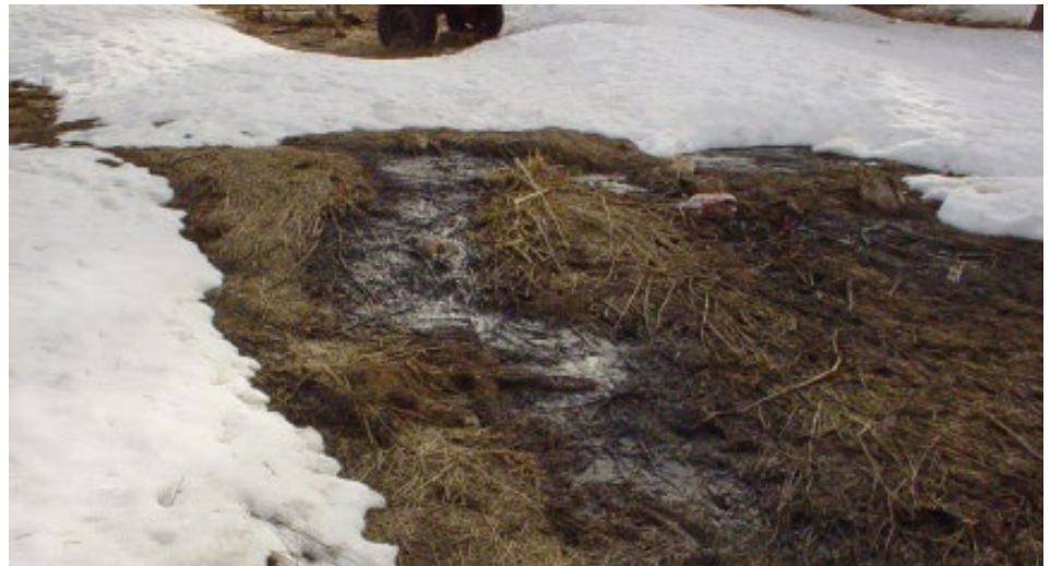
Commonly when a drainfield fails, effluent can be seen surfacing in the area.
