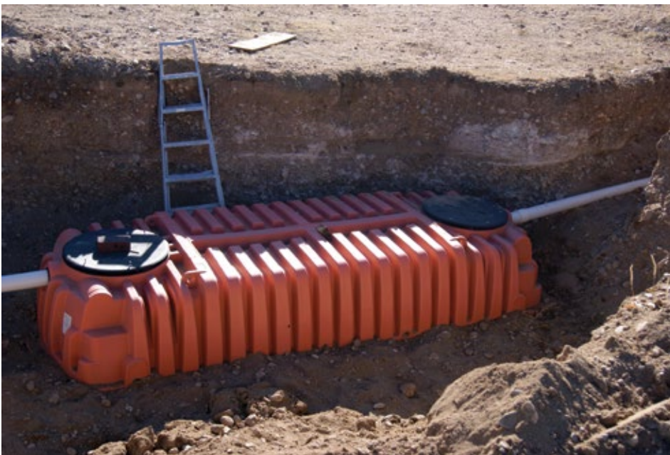
Gravity fed system in a trench configuration. A plastic (poly) tank and distribution box are used with this system.
