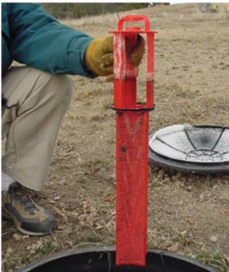
An effluent filter reduces the possibility of solids moving out of a tank and clogging a leach field.
