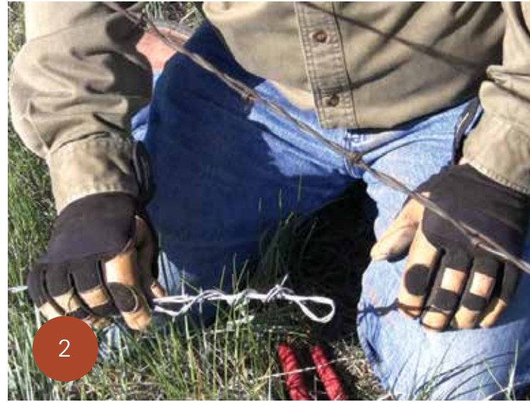
Build a loop in one end of the broken wire. Fold approximately 10 to 12 inches of the end back on to itself and twist it around the main wire four to six times. Repeat this step on the other end of the broken wire.
