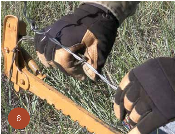
After the barbwire is tight, measure the patching piece of barbwire and cut with fencing pliers so that 12 inches or so extend from the stretchers. Next, insert the loose end of this wire into the loop on the existing fence and twist back on to itself four to six times.
