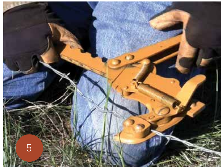
Ensure the stretcher is fully extended. Attach the end of the broken barbwire with the remaining single loop to one end of the fence stretcher. Hold up the non-looped end of the roll of patching barbed wire and estimate how long of a piece you'll need to complete the patch. Place this wire into the other end of the wire stretcher. Start ratcheting the fence stretcher and continue until the wires are taut. If you find that your estimate for the length needed isn't correct, release the stretcher, reattach the patching piece at a new part of the wire, and repeat the ratcheting process.
