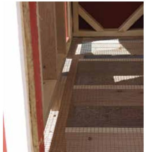
Turn base right side up and add the wheels. Cut to fit and attach the mesh screen to the base.
