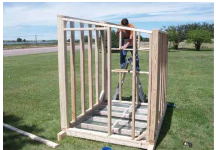
Complete the frames for end and side walls. Set walls in place. Attach walls to floor.
