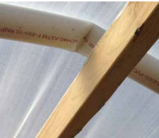
The snow load kinked this PVC rib around the center support of this high tunnel at Encampment. The PVC rib has been compromised suggesting the use of additional bracing to prevent the complete collapse of the structure and replacing ribs when a new cover is needed.
