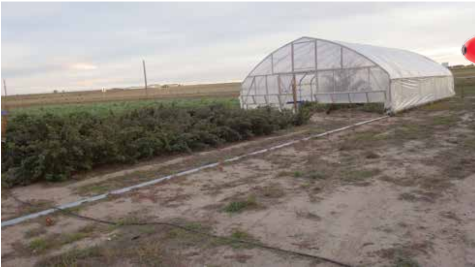
The high tunnel is on tracks and moved north or south to protect different crops at different times of the growing season.
