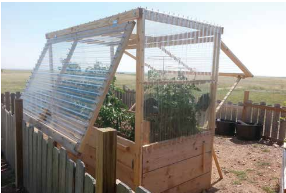
This mini-greenhouse-like structure in Christy Crochet's garden provides hail and wind protection and conserves some heat. The polycarbonate cover sustained no damage during a golf-ball-sized hail event last year.
