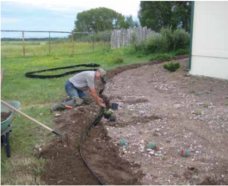
Installing the edging.
