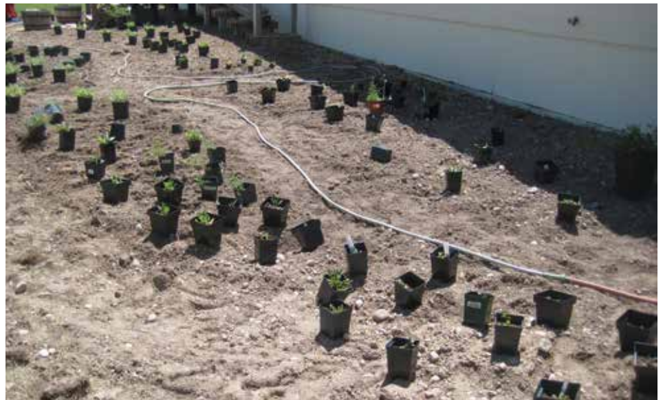
Plants have been placed where they will be planted.
