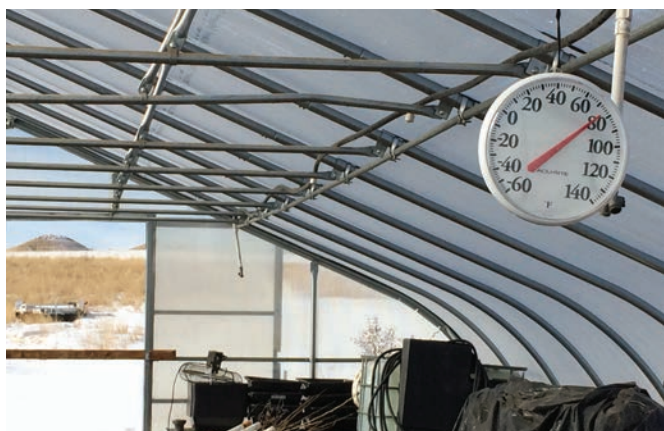
Doors have to be opened to work inside on warm sunny days.
