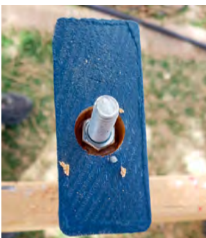
A hanger bolt that has been screwed and glued into the strut. The end you see will be placed through a drilled hole in the hub.
