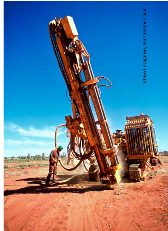
Drilling for core samples
