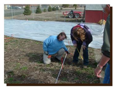
Along both lengths of the Hoop House and inside the string, drive 24 in. rebar stakes every 3 ft. apart, 12 in. deep, at 30 degree angles, until you reach the desired length.
