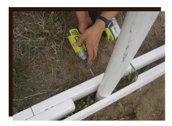
The outer baseboards should each be one 1 in. x 4 in. x 12 ft. and two 1 in. x 4 in. x 10 ft. boards, butted and fasted together by short (14 in.) brace pieces with the 12 ft. board in the middle. The inner baseboards should each be one 2 in. x 4 in. x 12 ft. and two 1 in. x 4 in. x 10 ft. Make sure the screws and brace pieces are facing toward the hoops when installing the baseboards.
