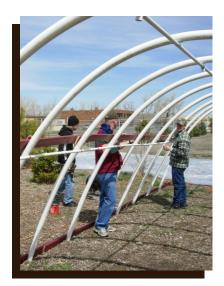
Mark the purlins every 36 in. where they will be attached to each 2 in. ribs. Two purlins will be attached 60 in. above the end of each pipe and one down the top middle of the hoop house. Marking the two end hoops and running s string can easily achieve a straight line.
