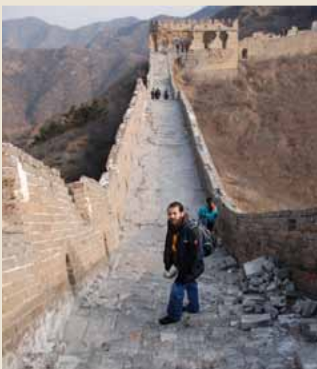
The Great Wall in Simatai
