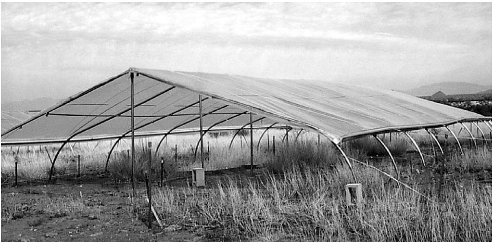
Fig. 1. Shelter (9 × 18 m, 4 m tall at apex) on the clay-rich site, open sides are > 1.5 m off the ground. Tall grasses visible beneath the shelter are H. contortus . Note the cables attached to the shelter and steel fenceposts for greater wind-stability and polypropylene rope holding down the plastic cover.
