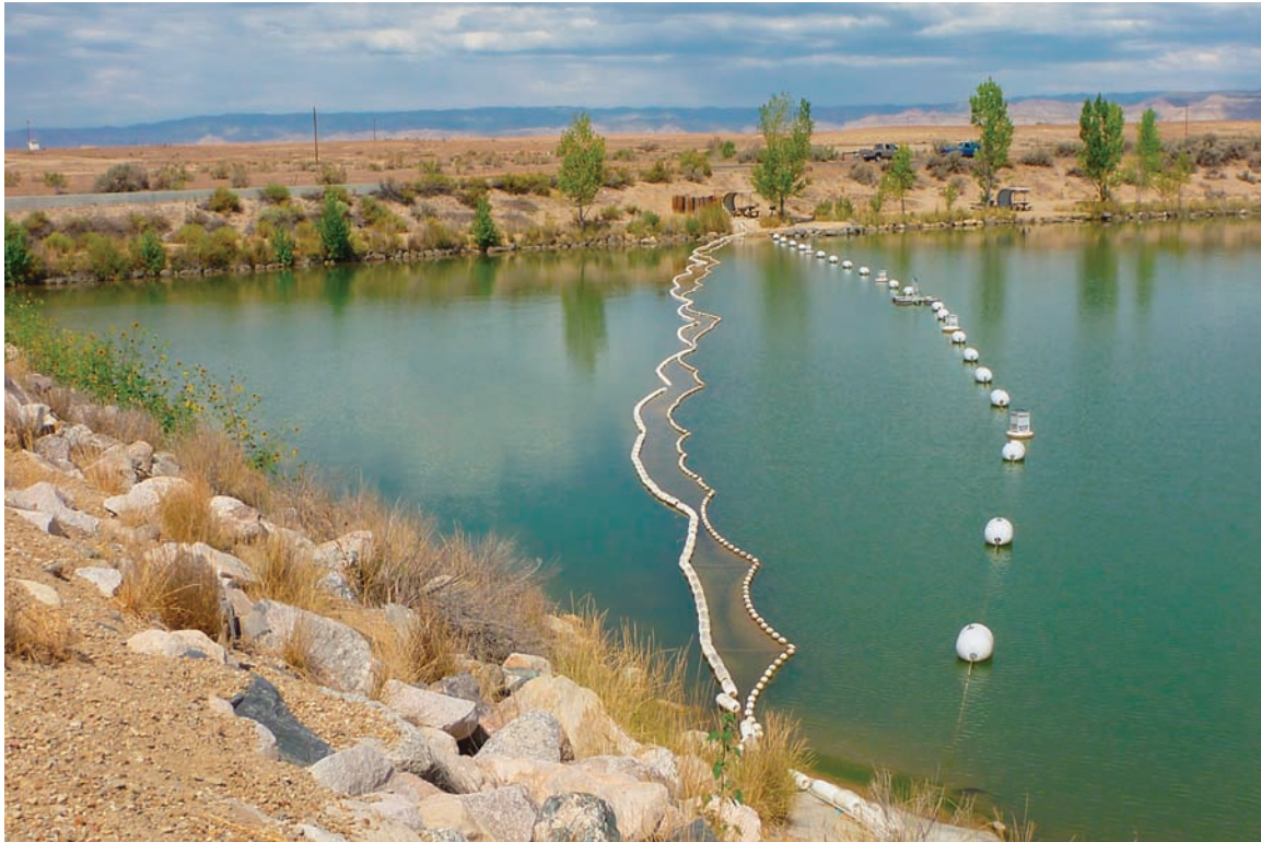
Figure 3. Net barrier in Highline Lake, Colorado, used to prevent the escape of nonnative sport fishes into an outlet stream that contains native fishes of conservation concern. Photograph: Danielle Tremblay and Jessica Hogue, Colorado Parks and Wildlife.
