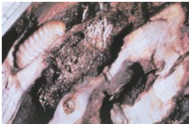
Photo 2. Borers and damage.
