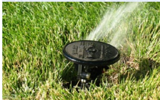
Pop-up impact sprinklers are commonly used in automated lawn irrigation systems.
