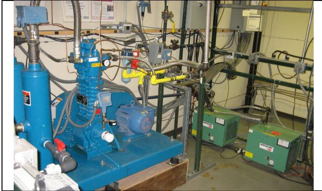
Figure 5. Low Pressure Compressor and Chillers
