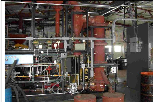
Figure 11. WRI Fluidized-Bed Gasifier
