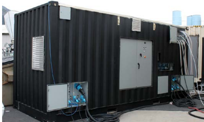
Figure 8. The coldbox container holds all 3 coldboxes and the cryogenerators. Hoses and cables connect the two containers.
