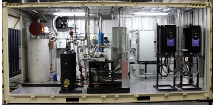
Figure 10. The pre-treatment container holds the flue gas pre-cooler, blower, and drier in the left half. The right half is dedicated to electrical control cabinets. Two large variable frequency drives can be seen on the right which drive the 60 horsepower cryogenerators.
