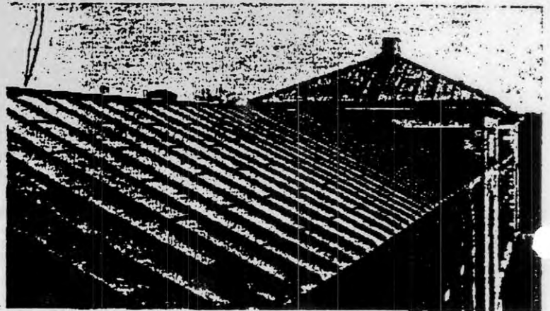
FIG. 5.—Building at Saratoga Springs, N. Y., with Lead Roof.
