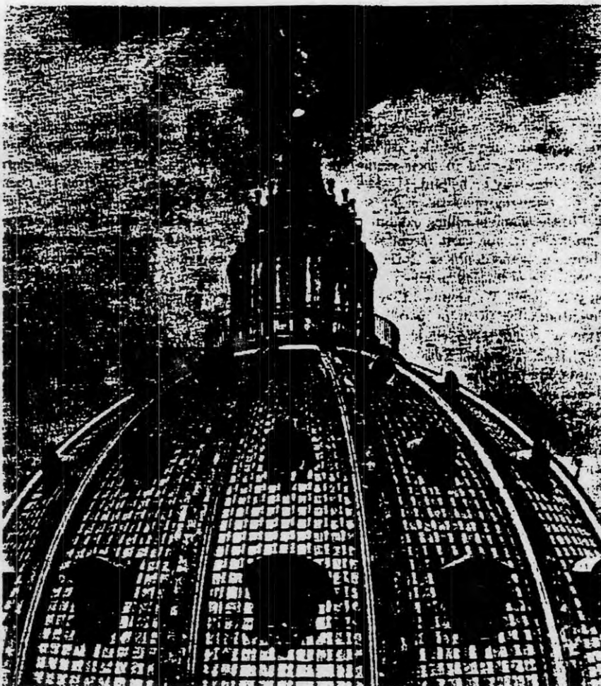
FIG. 7.—State Capitol Dome, Harrisburg, Pa., with Lead Ribs and Lantern Totally Roofed with Lead.
