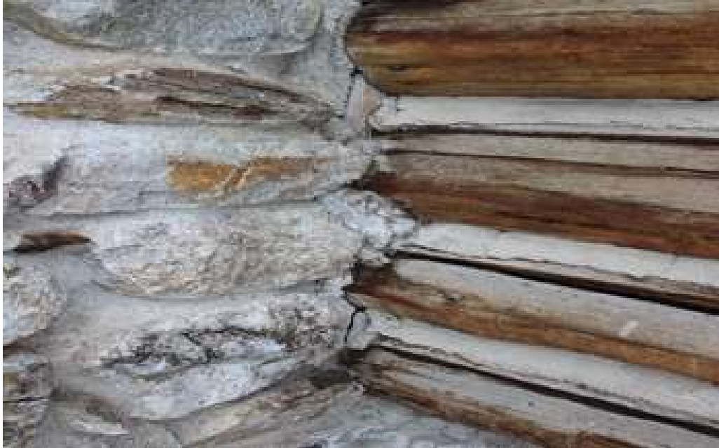
Johnson Lodge, insulation needs to be replaced and the exterior of the building sealed using chinking and sealant.
