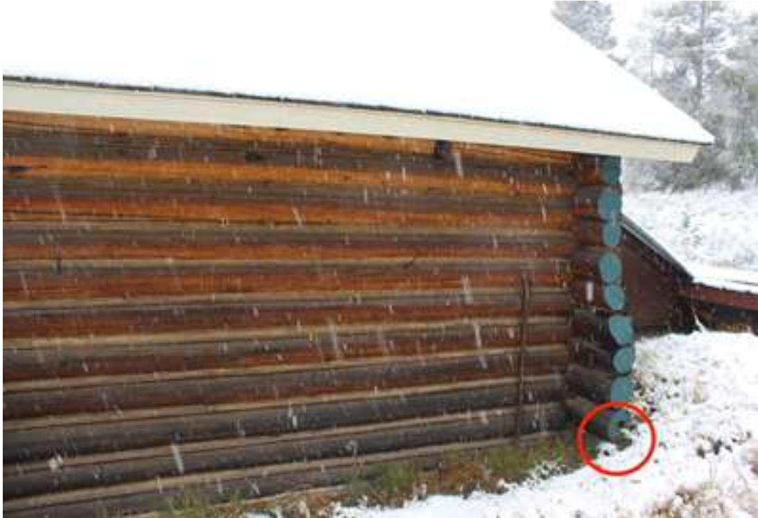
1 log-end needing replacement.
