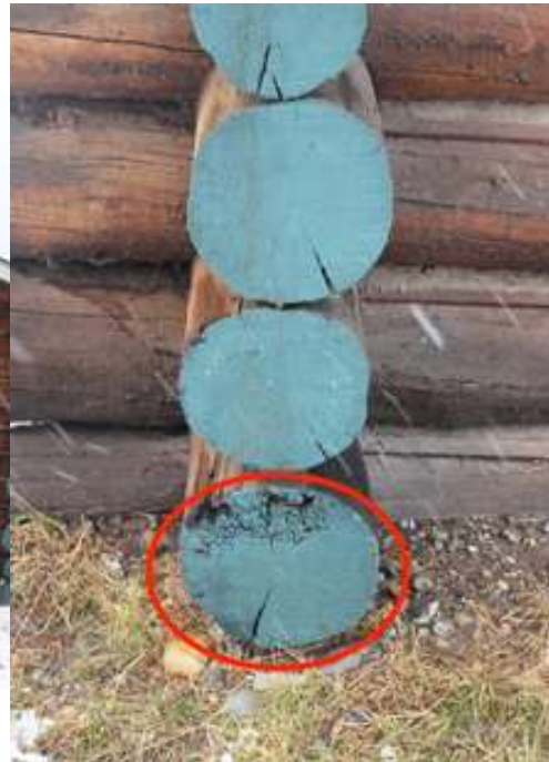
Replacement of 7 log ends and one horizontal log. Boat house, backside with close up of logs that need to be replaced on the north side. Arrows point to horizontal log that needs replacing, see close up.
