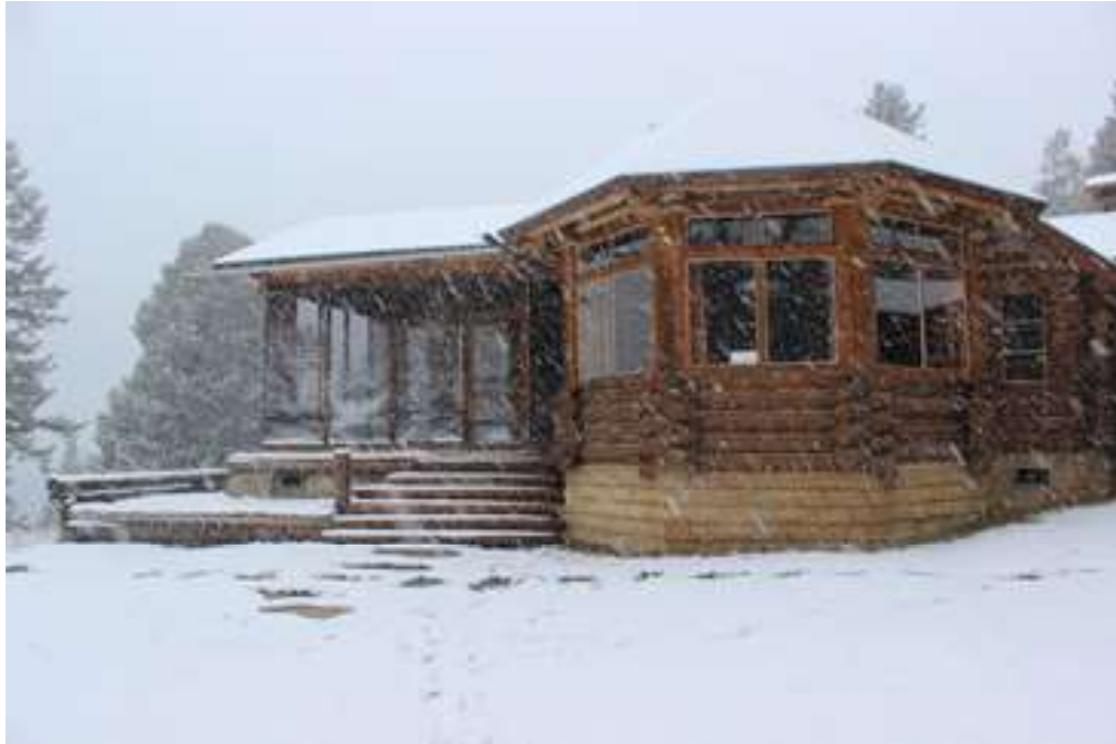
View of Berol Lodge at the exterior enclosed porch. The porch structure has deteriorated and is unlevel due to ground conditions. Much of the exterior exposed structure, floor boards and some vertical columns show wear and degradation. These elements need to be replaced in-kind to maintain the historical look. The screening enclosing the porch also needs some attention.
