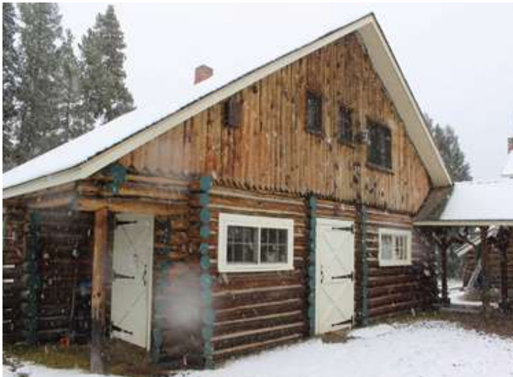
Johnson Lodge garage building. 3 log ends and one post that need replacing, see close-ups.
