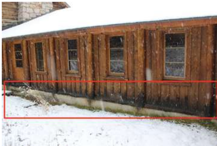
View of the north side of the building. Here is an example of snow damage to logs, turning them black at the bottom of the exterior walls. This is suspect of mold and should be cleaned by pressure washing, stained and resealed.
