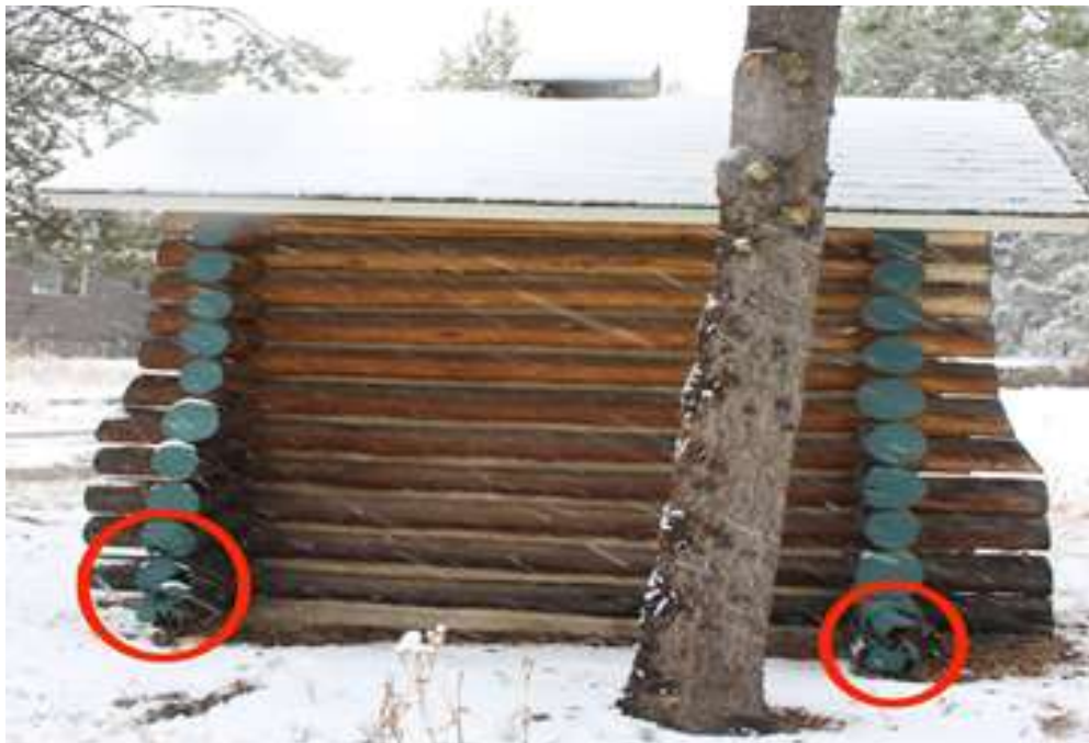
Cabin - right side of front, 5 log ends needing to be replaced.
