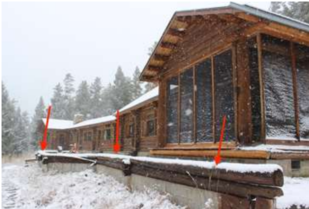
View of the south face of the building and screened porch. The log fence around deck needs to be replaced, see close-up photos in next view.
