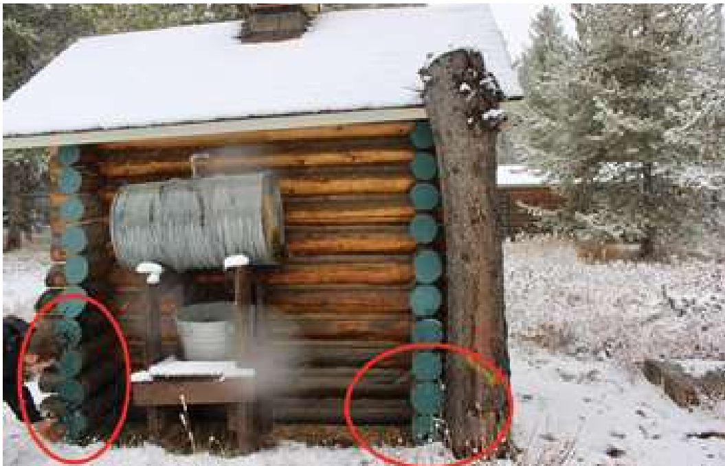
Cabin ??, replacement of 6 log ends on left side of front.
