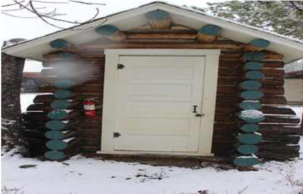
Cabin, front view - replacement of 11 log-ends.
