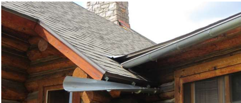
Roof & Gutter Improvements
