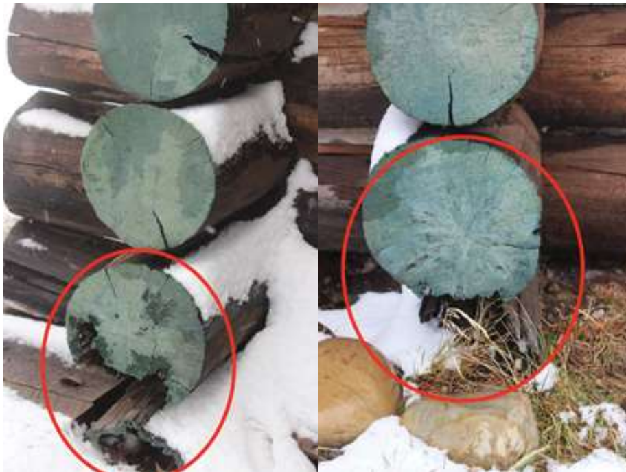
Boat house, right east side, front, 3 logs needing replacement.
