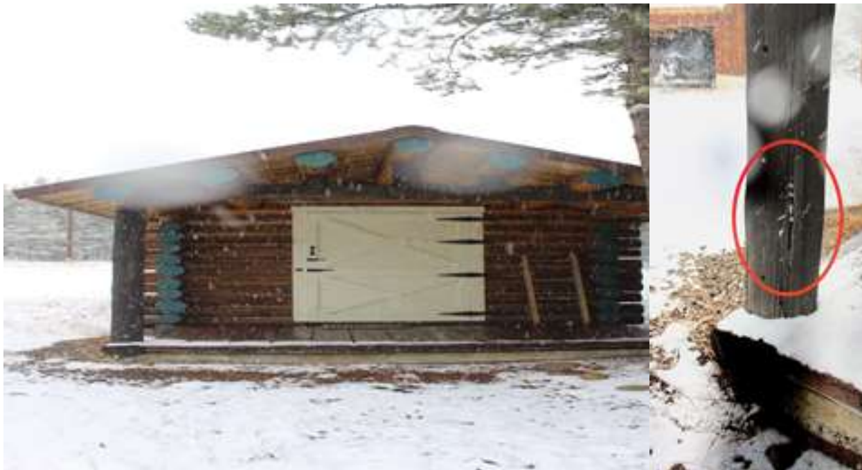
Cabin No. 1356 Replacement of 1 log on front deck, see close-up. And re-think some spots. Cabin no. 1356, column log on front deck needs to be replaced.
