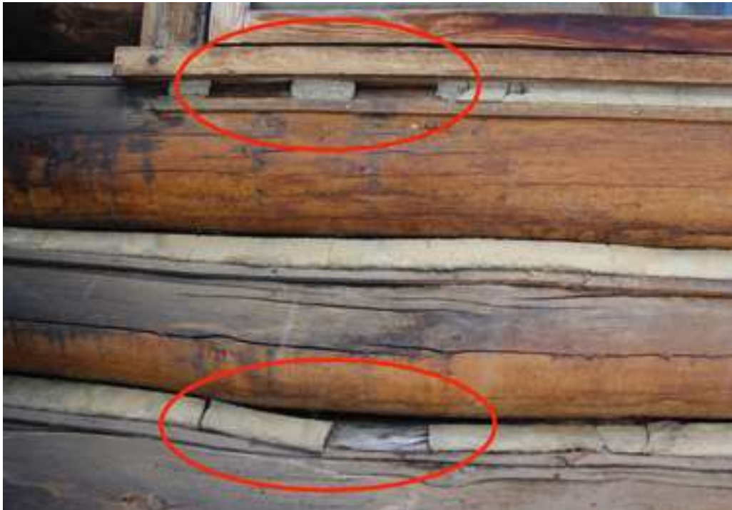
Johnson Lodge, insulation needs to be replaced and the exterior of the building sealed using chinking and sealant.
