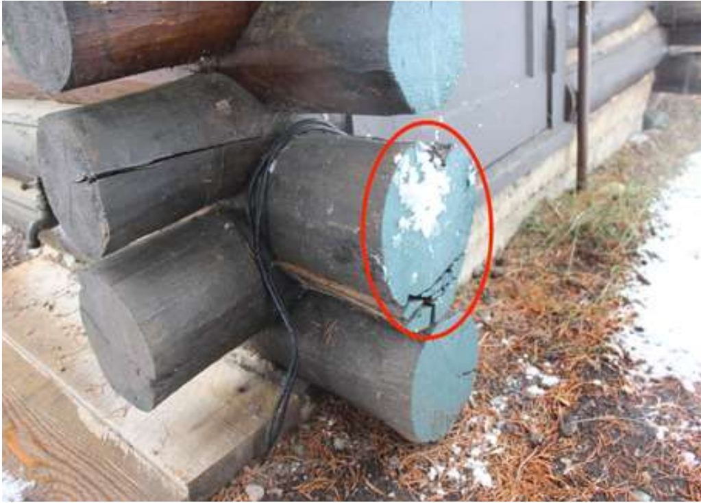
Close-up view of an example of building log-ends that need replacing.
