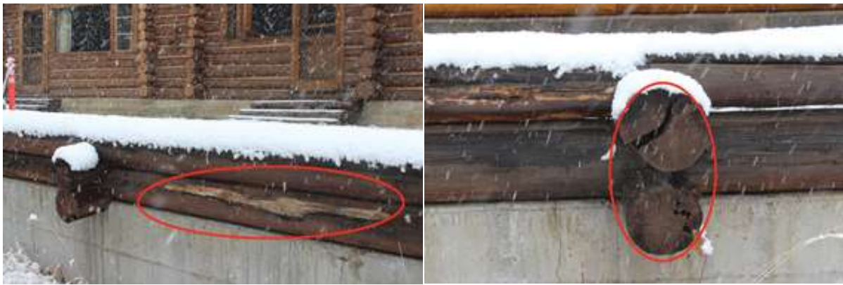
Examples of damage on the fence around the deck.
