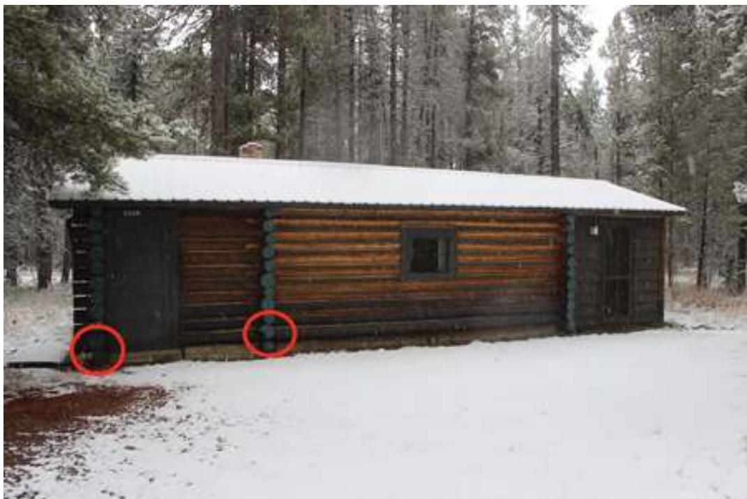
2 log-ends that need replacing on left side of front.
