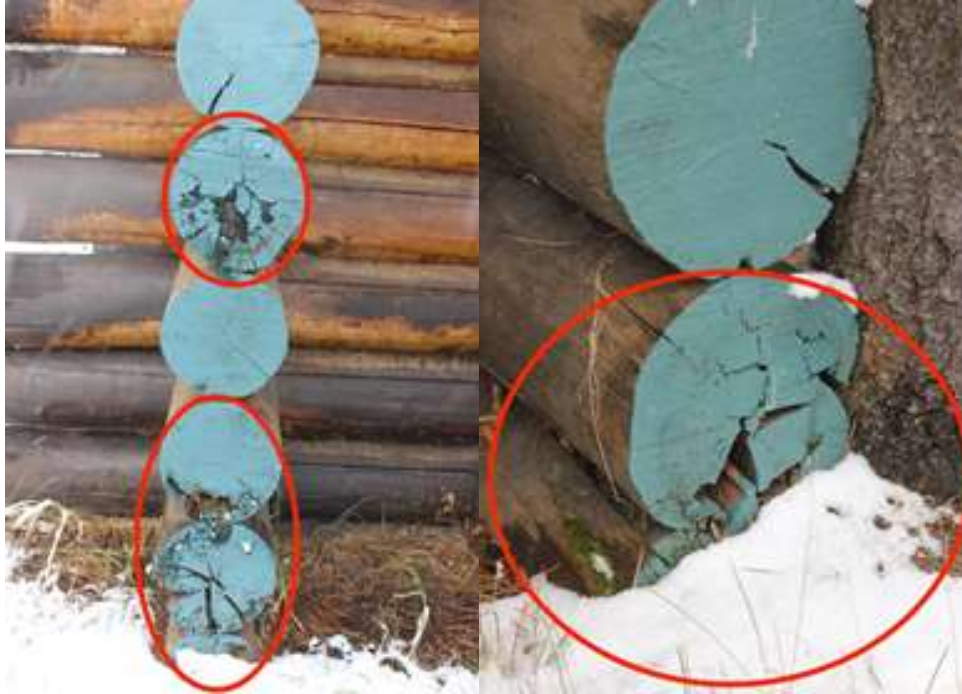
Cabin - close up of log ends needing to be replaced on left side of front.
