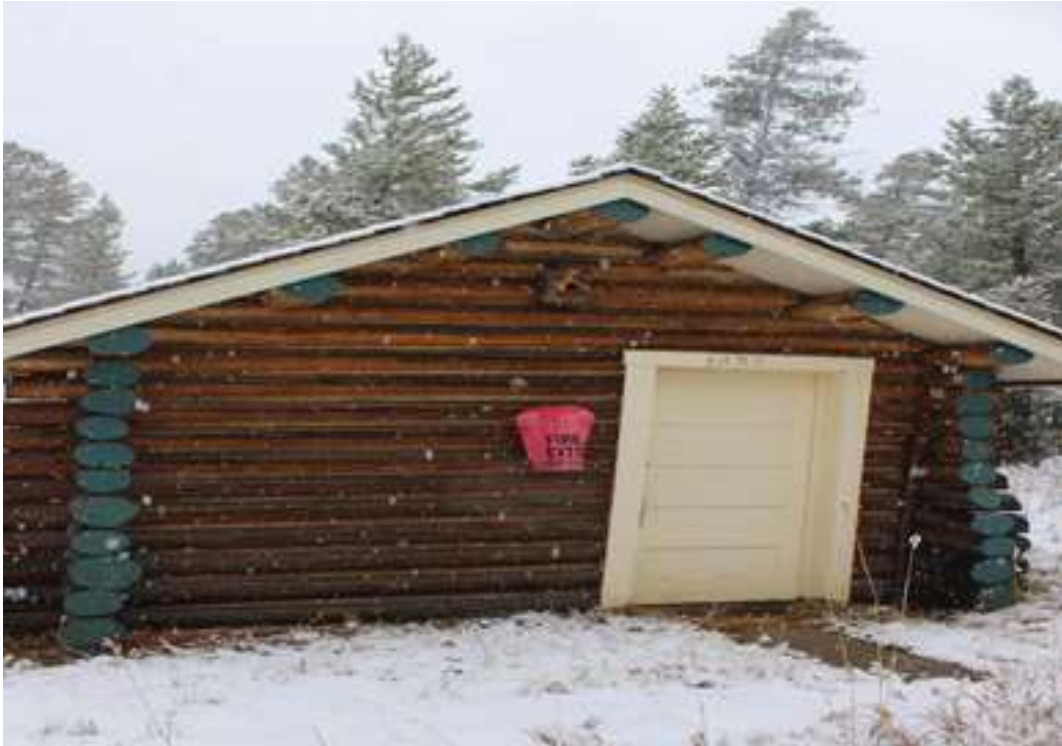
No. 1353 - Replacement of 3 log ends, left side of front.
