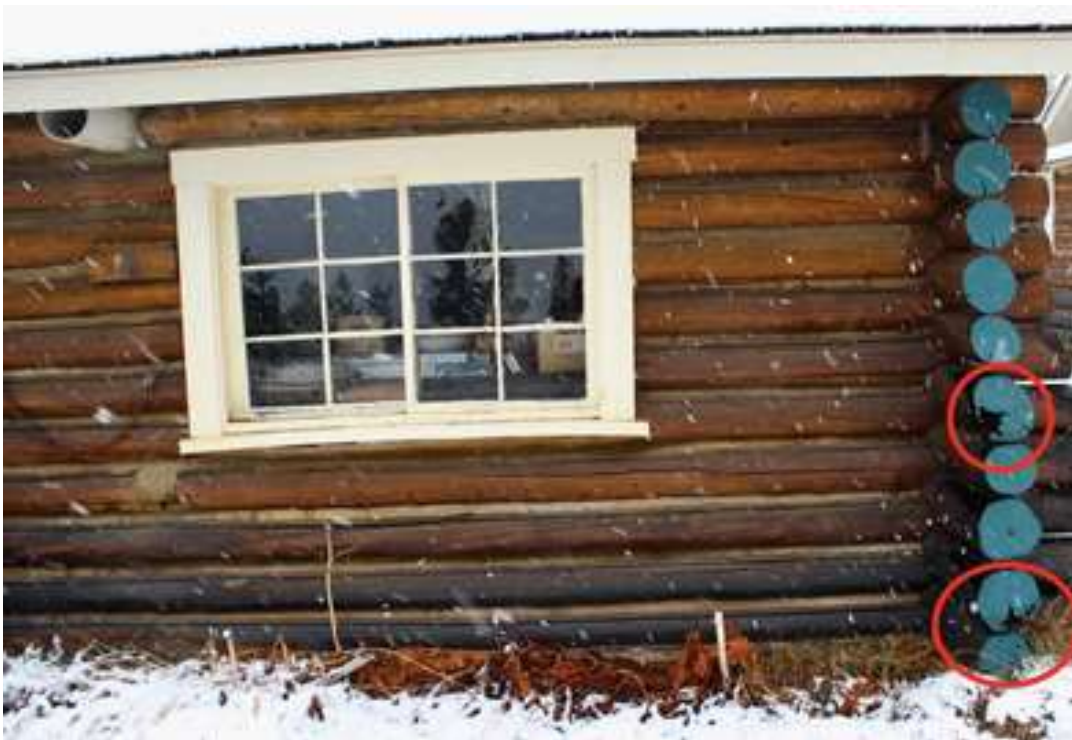
Cabin no 1353, 3 log ends that need replacing on left side of front.
