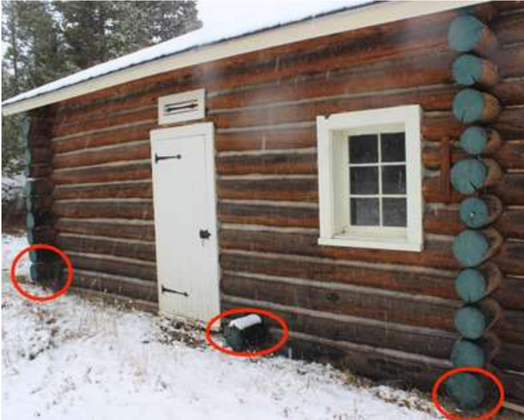
Boat house west side front, 3 log ends need replacing
