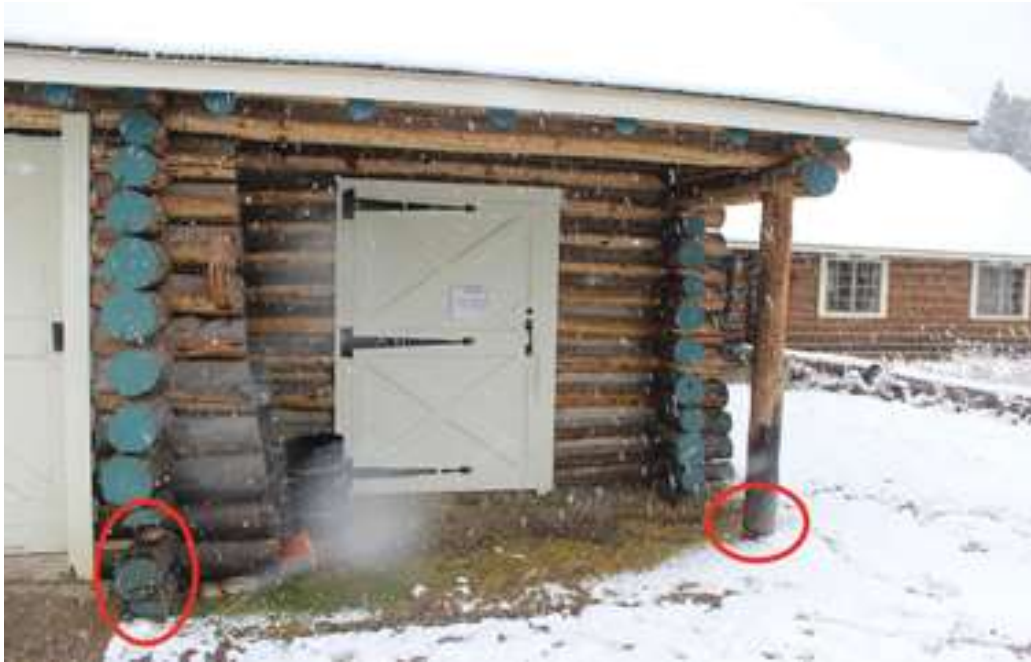
Example of spot that needs re-chinking.
