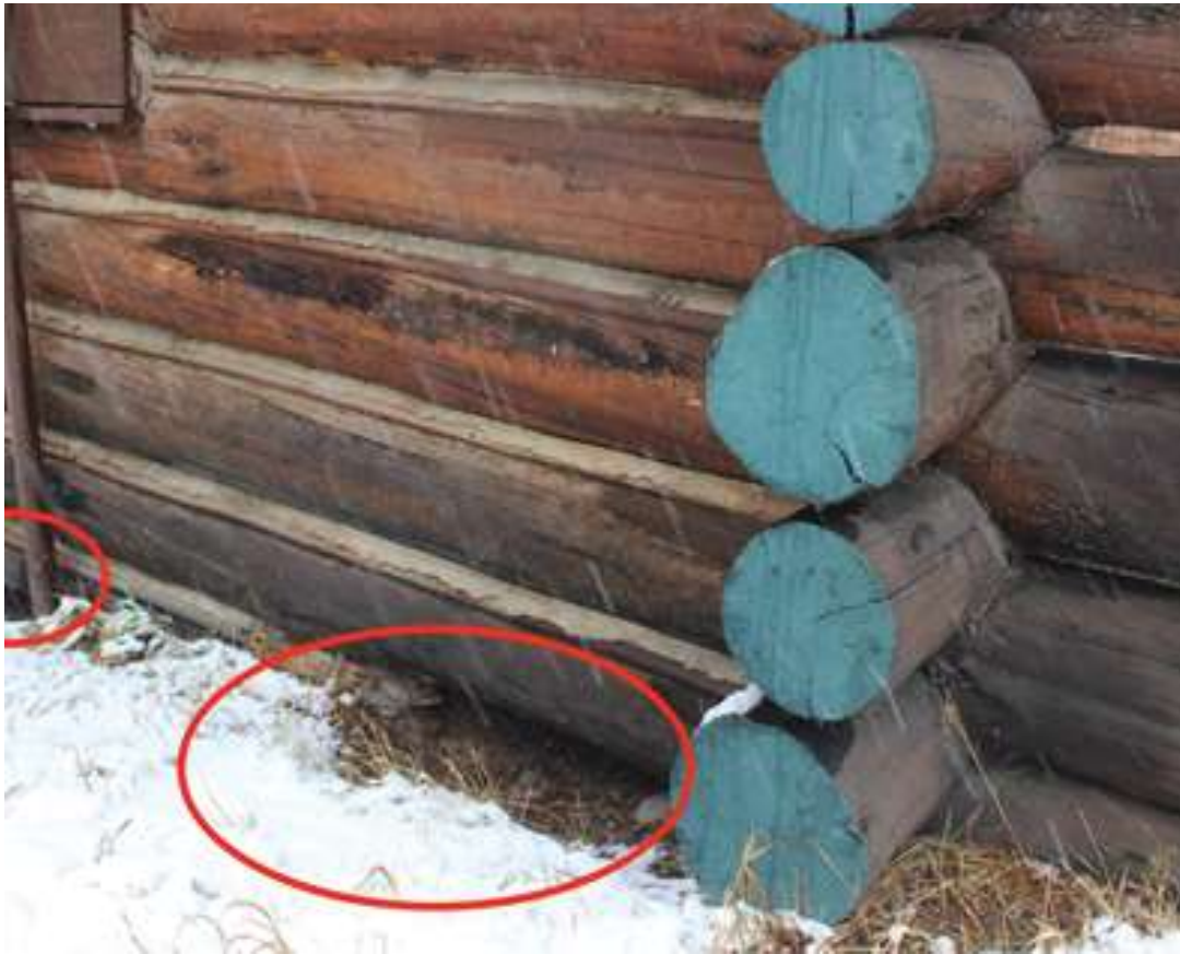
Boat house, back side, close-up of horizontal log needing replacement.
