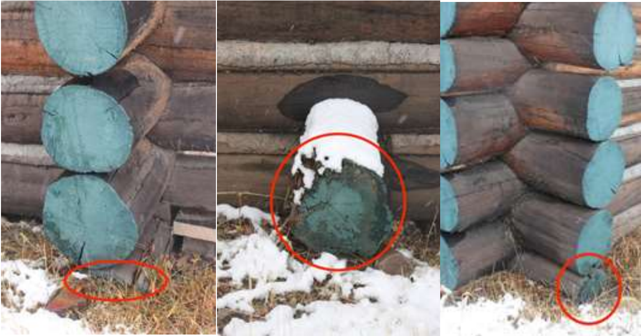
Boat house, close up of 3 logs needing to be replaced on left side of front.
