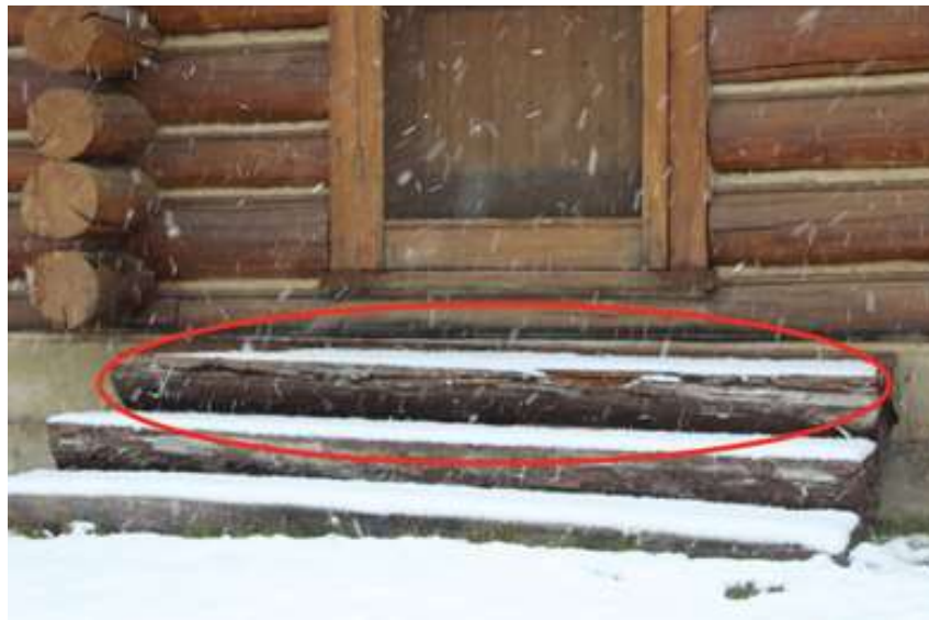
Exterior step that needs to be replaced. The grounds crew have replaced on set of stairs on the west side, and the work is well done and matches the historical for the building.
