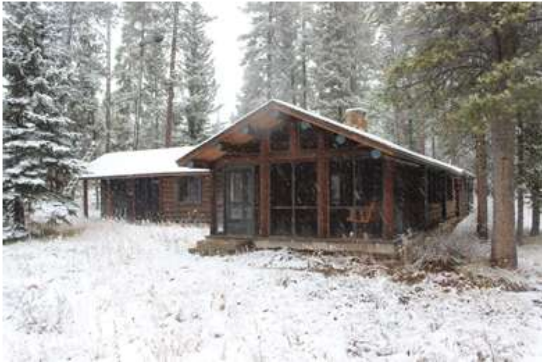
Replacing 2 log ends on the left side of front, see close-ups. South view
