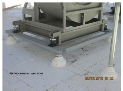
LARGE ROOF FAN FLASHING
