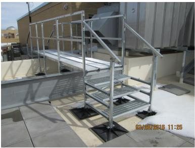
ROOF WALKWAY & STAIR WITH NON-PENETRATING BASES
