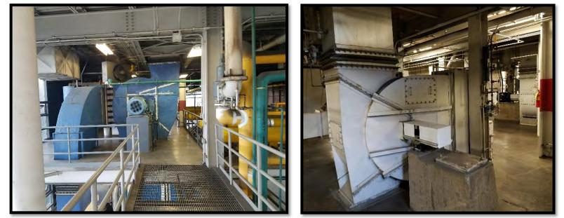
ID Fan: 150 HP, 1192 RPM, VFD present. South ID fan: VFD does work. Harmonic Guard Power conditioning is suspect. Center ID fan: Clarage Fan, manufactured by Air Systems, Kalamazoo, MI. Serial No. 2696CM-5. Size 132, type XLR, series 1250. 1200 Max safe RPM at 430°F.
