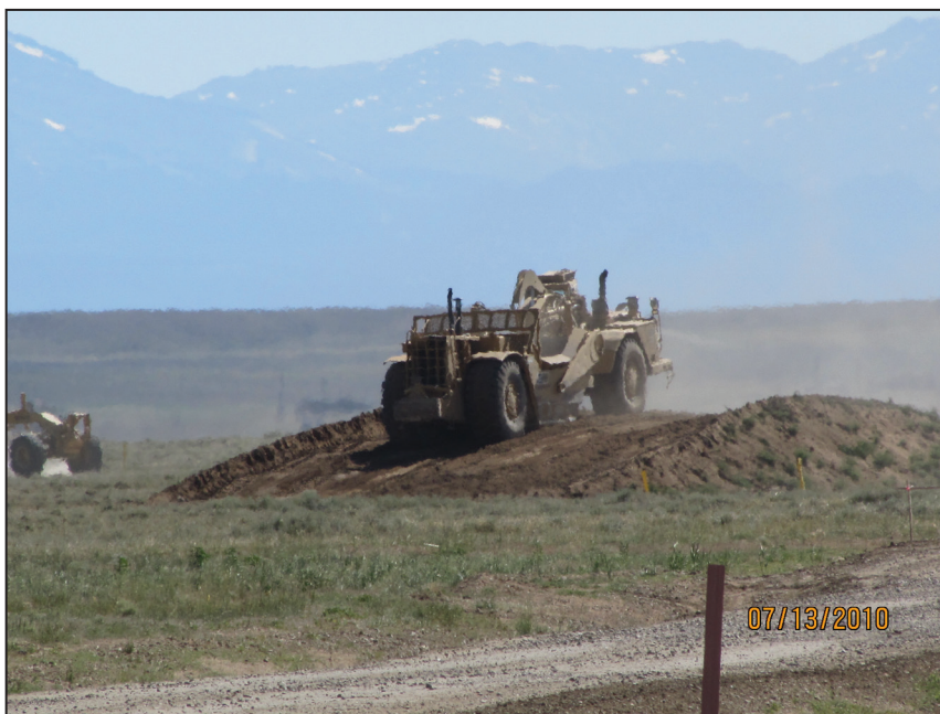
Respreading topsoil
