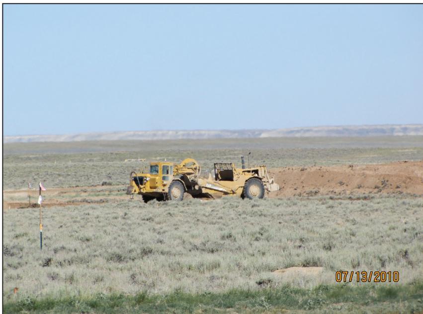
Stripping topsoil
