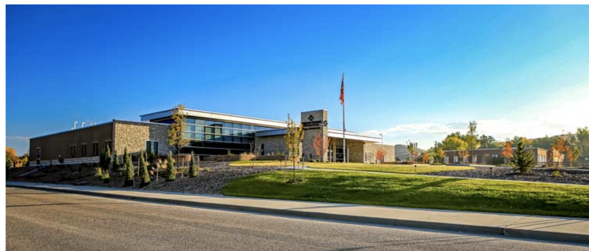
Memorial Hospital of Converse County - Medical Office Building: Location of Primary Care Services for Douglas and tri-county area
