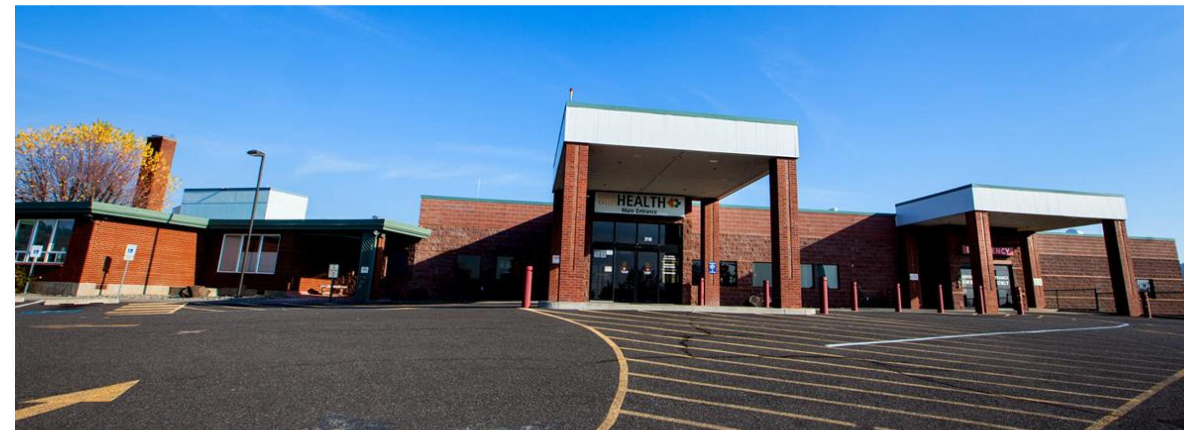
Klickitat Valley Health Main Entrance
