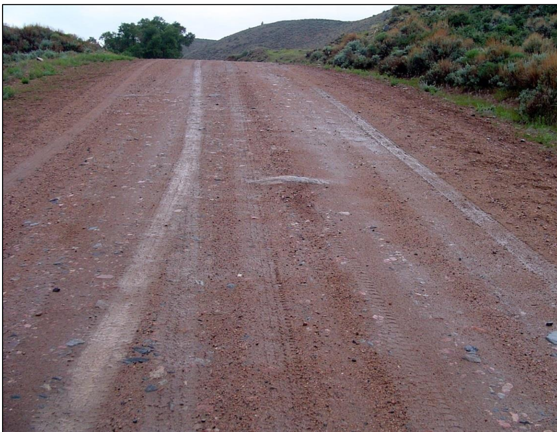
7 – Good 40 - 45 mph Significant roughness, distresses and loose aggregate.
