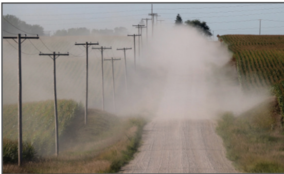
Dust poses a hazard for workers and motorists. (Source: Soil Stabilization of Oklahoma).
