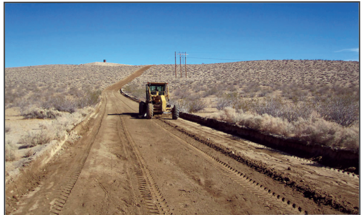
Grading is the primary maintenance performed on unpaved roads (Source: Envirotac).
