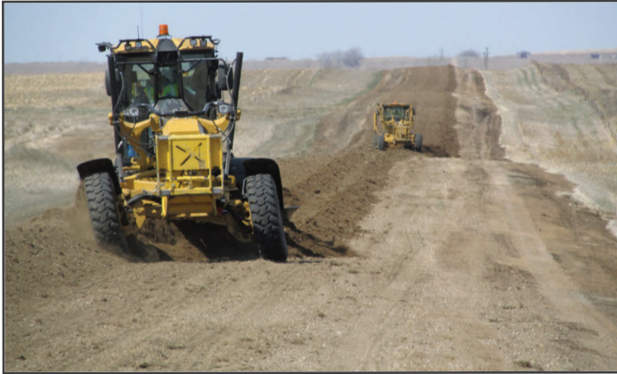
Reconstruction work space. (Source: Greg Vavra, SDLTAP).
