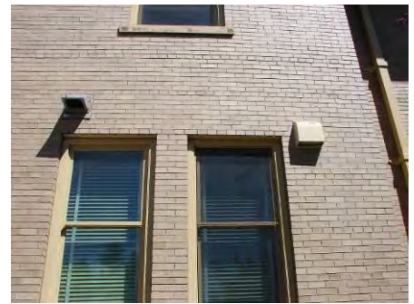
Limestone details showing open joint, chipping, and surface spalling; replacement windows and vents in brick masonry
