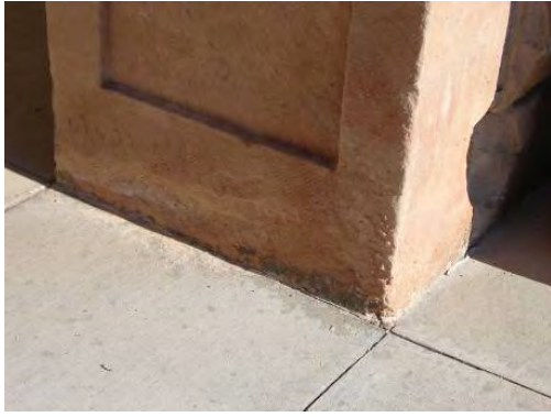
Surface spalling at entranceway; cracking at stone spandrels
