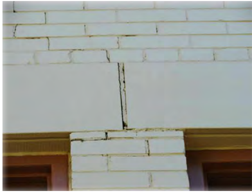
Cracks at lintels due to jacking
