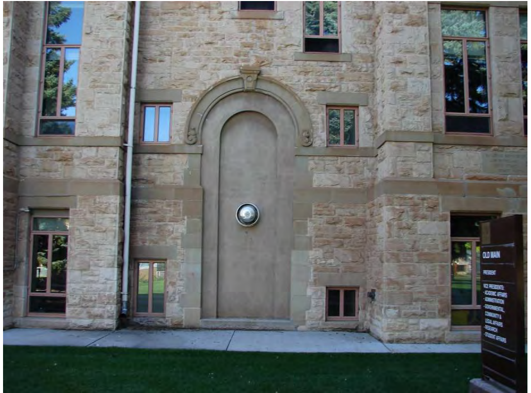
Unfortunate stucco infill at former secondary entrance, west elevation.
