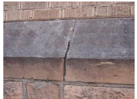
Cracked joint at window sill; west elevation with metal plates; open joint in watertable, west elevation
