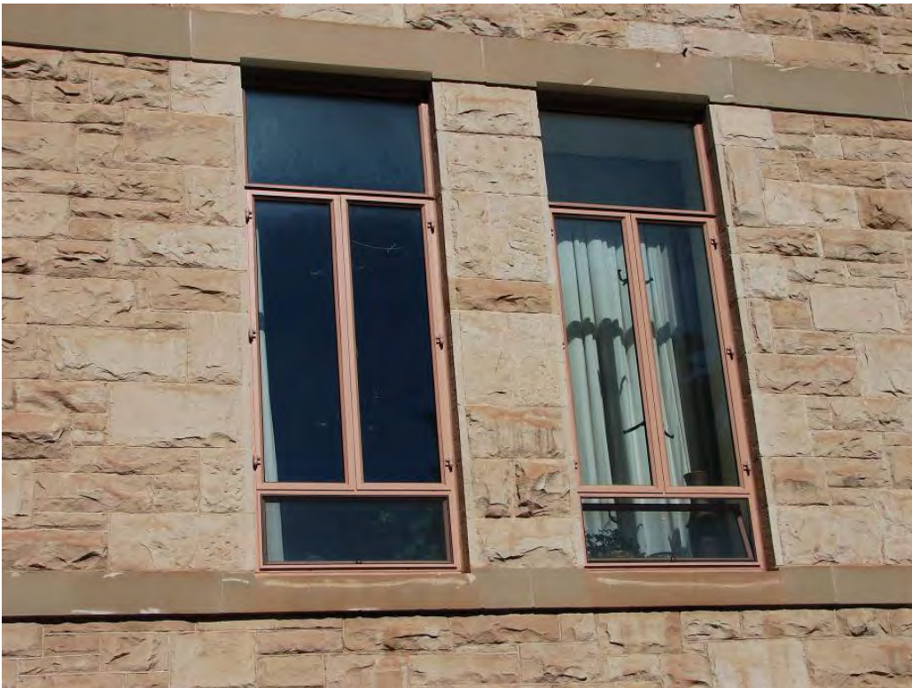
Original windows were wood doublehung with a decorative transom at the top. These 1949 replacement windows are metal casements with a hopper at bottom.
