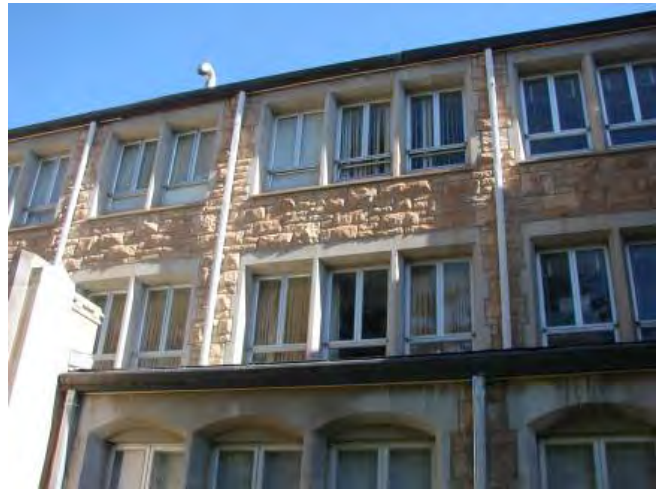
Stone detailing and infilled windows of Science Hall, details of the 1954-56 addition
