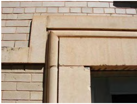
Limestone details showing open joint, chipping, and surface spalling; replacement windows and vents in brick masonry
