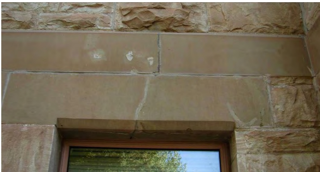
Cracking of dressed stone at joints and through the stones; surface deterioration as well.
