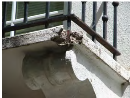
Masonry, concrete, and stucco deterioration due to water penetration
