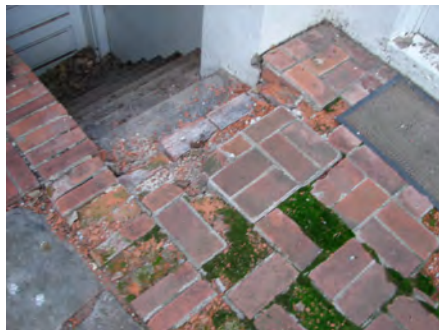
Masonry, concrete, and stucco deterioration due to water penetration
