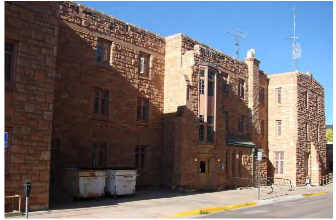
South wing showing vertical joint between the original 1941 building and the 1950 addition; north elevation showing the entrance that originally faced Prexy's Pasture
