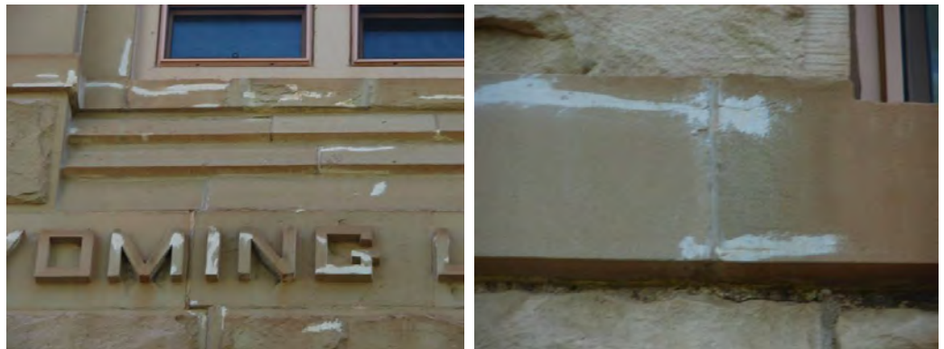
Poor joint repairs have created an unsightly appearance.
