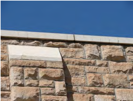
Fine cracks in pilaster and parapet caps, and minor cracking of mortar joints in stone walls
