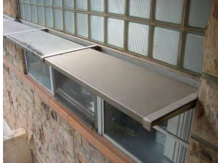
Entrance of American Studies wing and details of windows and aluminum sunscreen
