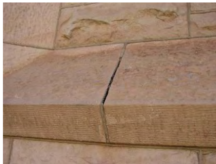
Vertical crack between windows, open joint in sloping watertable, detailing of stone entranceway of Science Hall
