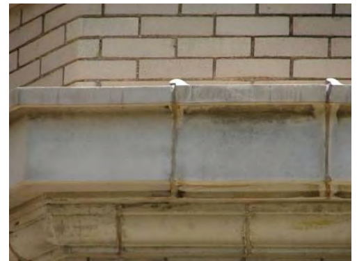
Joint that has been etched by cleaning and repaired with sealant; covered top joint
