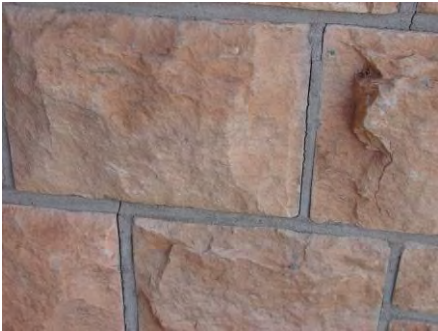
Fine cracks in pilaster and parapet caps, and minor cracking of mortar joints in stone walls
