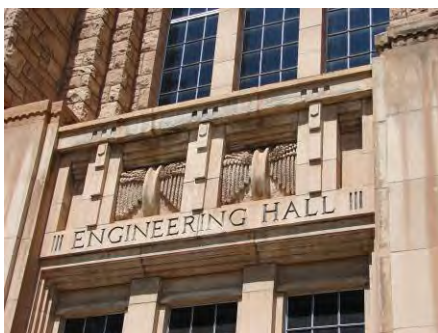
Weathered detailing at top of entrance; original metal windows of Engineering Hall (left) and the Petroleum wing (right)
