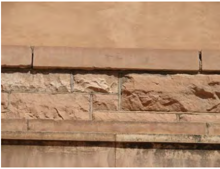
Open joints in masonry; view of 2015 east addition under construction
