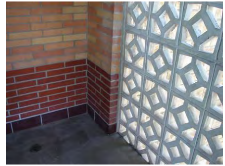
West entrance flanking lobby/café, original aluminum window, concrete block screen in open exit stairway
