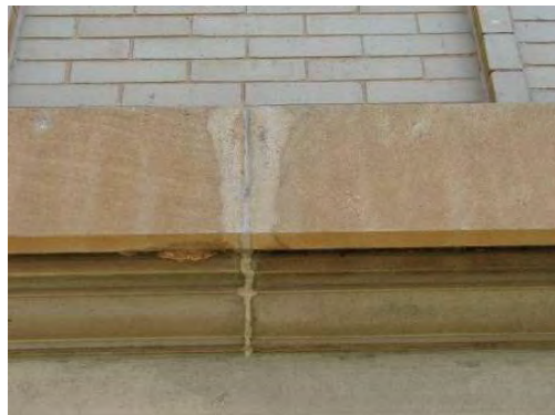
Joint that has been etched by cleaning and repaired with sealant; covered top joint
