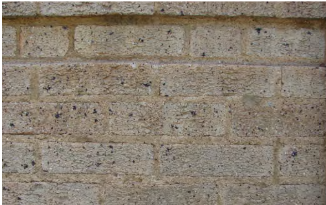
Rough/high textured wire cut brick on Aven Nelson
