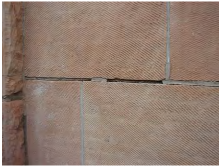
Missing mortar in spandrel panels and at a vertical wall joint
