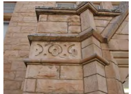
Vertical crack between windows, open joint in sloping watertable, detailing of stone entranceway of Science Hall
