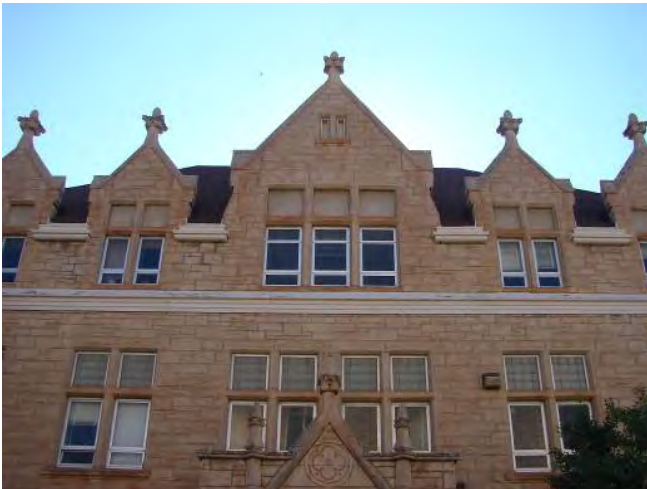
Stone detailing and infilled windows of Science Hall, details of the 1954-56 addition
