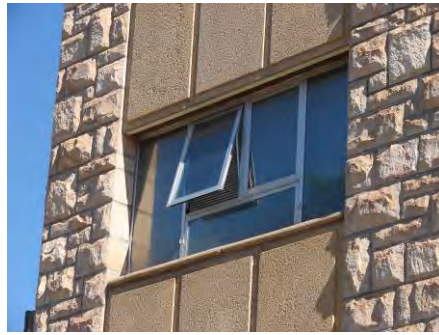
West entrance flanking lobby/café, original aluminum window, concrete block screen in open exit stairway
