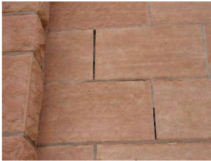
Missing mortar in spandrel panels and at a vertical wall joint
