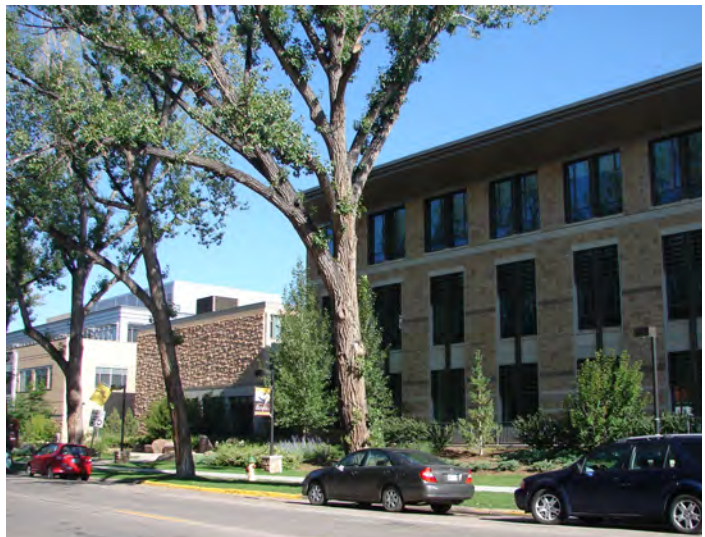
Large overhang for shading on Business Building
