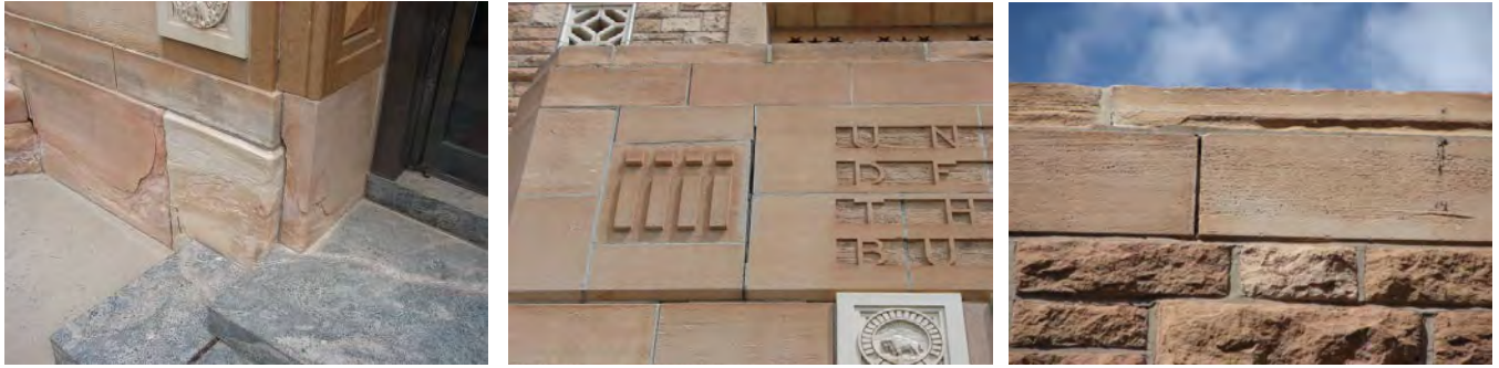
Delamination of base stones at entrance; open joints in stonework over entrance and at parapet
