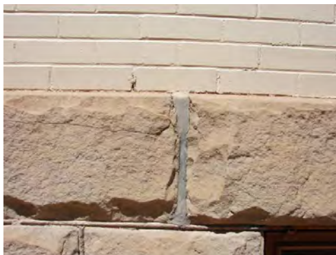
Inappropriate repairs with grey mortar
