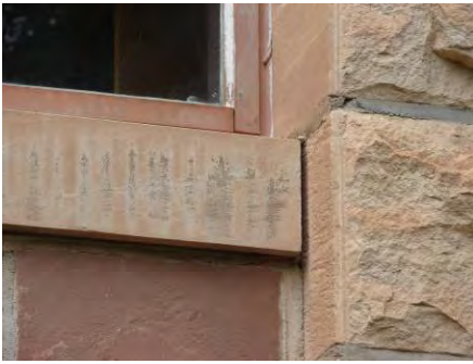
A few locations with open mortar joints.
