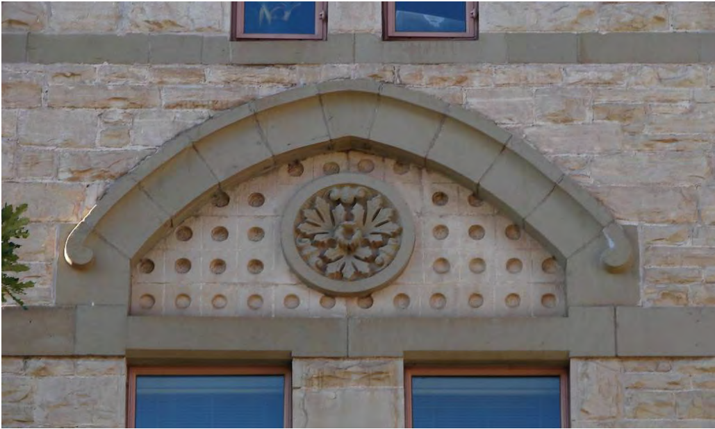
Fine stone detailing on the north elevation. Some joint repair is needed.
