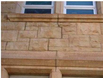
Vertical crack between windows, open joint in sloping watertable, detailing of stone entranceway of Science Hall
