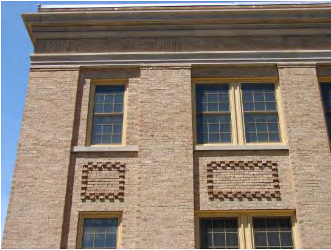
Masonry details and replacement windows; Brick repair with poor color match
