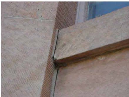
Cracked joint at window sill; west elevation with metal plates; open joint in watertable, west elevation
