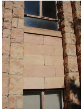
Surface spalling at entranceway; cracking at stone spandrels
