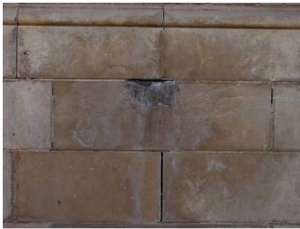
Limestone details showing open joint, chipping, and surface spalling; replacement windows and vents in brick masonry
