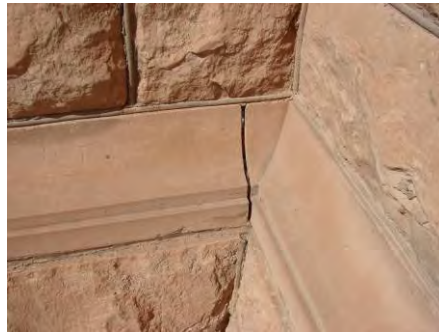
Open joints in masonry; view of 2015 east addition under construction
