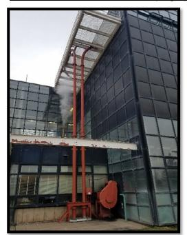
From truck dump, coal is transferred to the Denseveyor Pot in basement. This can blow to the silos or dry storage. Silos are along outside wall, 3 present. Dry storage is boiler specific. East pot is from truck dump.
