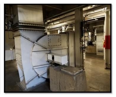
No. 3 Overfire Air Fan: Buffalo, Shop order number N2345. 26" wheel diameter, Size 7x26, Type E, 50 HP. No. 4 Overfire Air Fan: Buffalo, Shop order number N2345. 26" wheel diameter, Size7x26, Type E, 50 HP.
