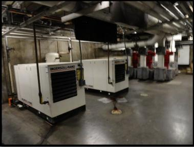
There are many uses around campus for compressed air. These include pneumatically actuated valves/positioners as well as various needs for the boiler system. There are several locations around campus where pneumatic power is generated including the CEP as well as Engineering Addition. New compressors are being installed as part of the new West Campus Satellite Plant.
