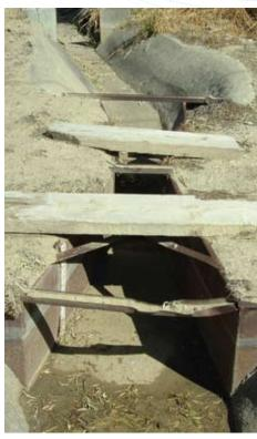
A simple concrete weir with gauge measures water flow.
