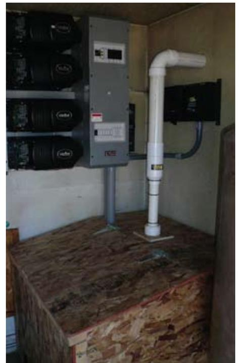
*An off-grid power system on a ranch near Farson. The battery enclosure is at bottom, with four 3,000-watt inverters on the wall, with solar and wind power controls on the wall at right.*
