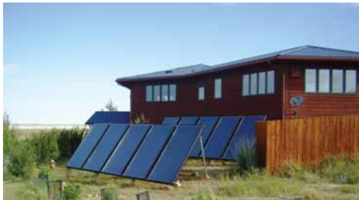
Figure 3 – An indirect circulation flat plate collector system.
