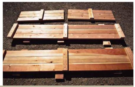
clamp together so ends are straight. Cut support piece to appropriate length (approx. 16") and screw for trellis) Cut (1) 2x4x5' and screw into place. Repeat steps 5&6 for opposite side.
