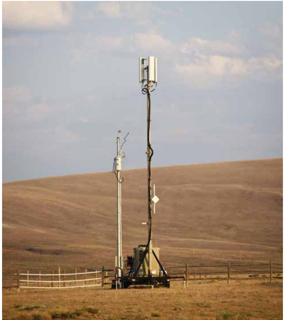
Modular cellular tower in Wyoming.
