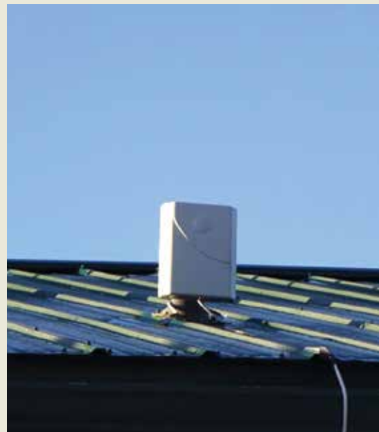
The outside amplifier is aimed at a cell tower to receive the signal.
