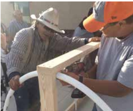
Figure 2. Attach the ribs to the 2x4 frame using 2-inch screws. The PVC ribs help support the plastic covering.
