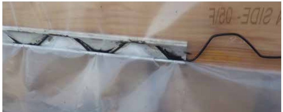
Figure 3. The wiggly wire helps secure the plastic and can be released to move the plastic covering up or down.
