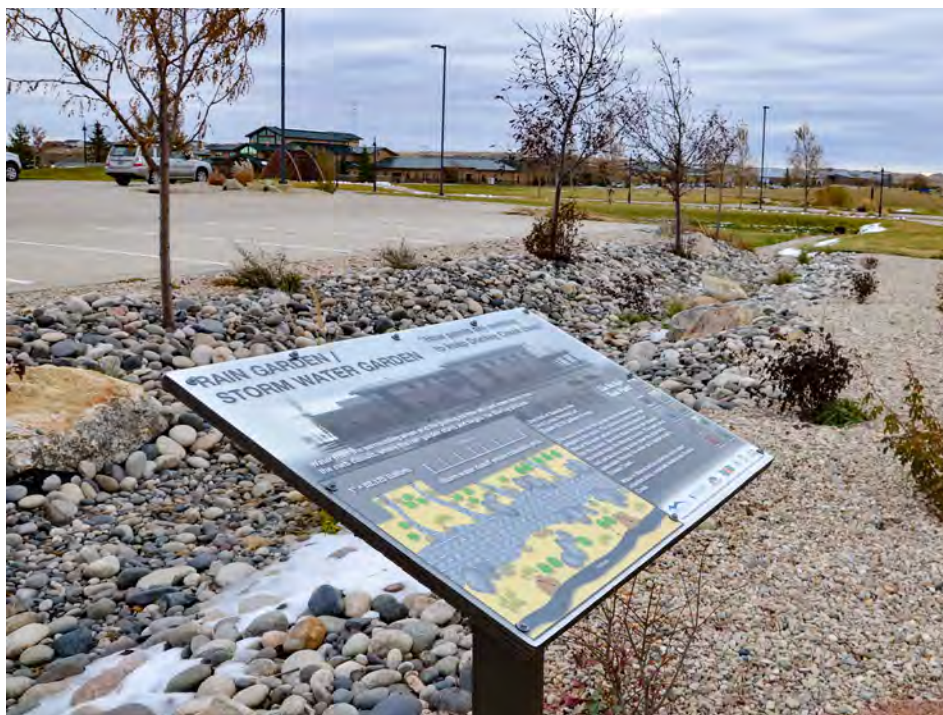
The rain garden adjacent to the Gillette College Technical Education Center collects runoff from the parking lot and filters contaminants before entering the Donkey Creek watershed. This view is looking downstream of the rain garden toward Donkey Creek. (Photo by Fred Harrell, NRCS-Wyoming public affairs specialist)
