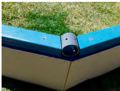
A dome connector (grey hub). The threads of the metal hanger bolt in the strut pass through one of the drilled holes of the hub and are attached using a Nylock nut.
