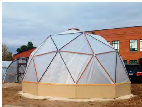
Completed structure in the Casper Veterans Garden.
