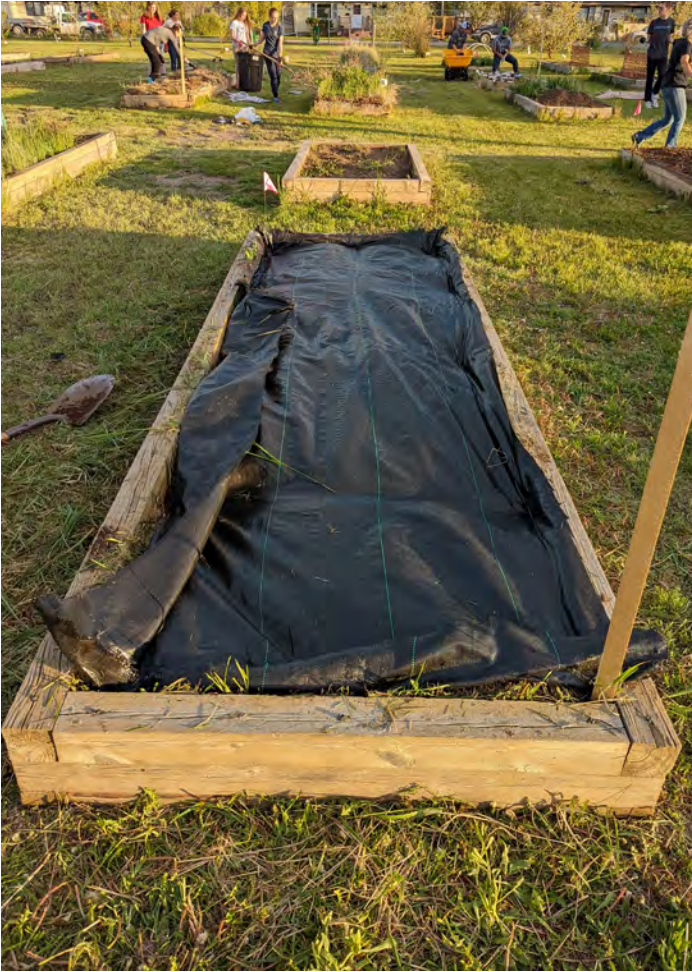
Installation of black landscape fabric in progress.
